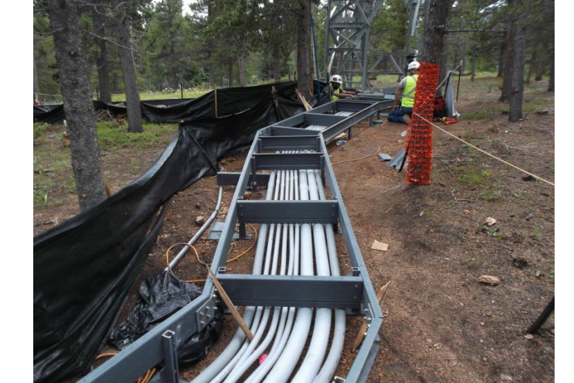
Figure 13. Boardwalk at CASTNET within construction limits; photo taken by construction supervisor
