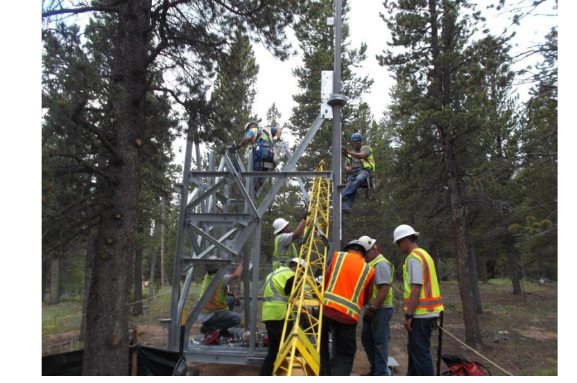
Figure 14. Contractors building tower at CASTNET; photo taken by construction supervisor
